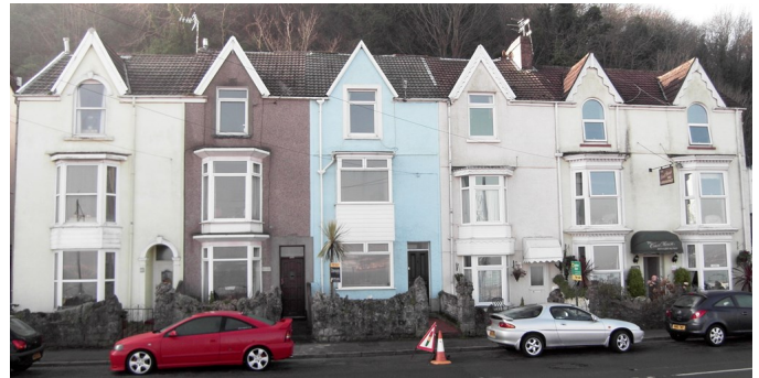
This attractive sea front terrace of Victorian houses displays the concerns of gradual change: loss of chimney stacks and pots; replaced gable barge boards; the removal of the arched top floor window openings; two inaccurately rebuilt two storey bays; changed window fenestration; door openings and doors have been replaced; and the pebble-dash wall finish does not respect the traditional design.
